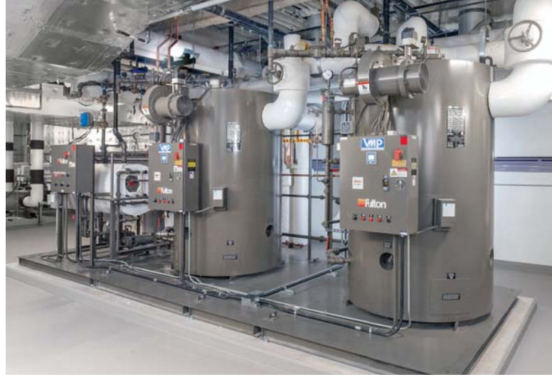
▲ A healthcare facility in Wisconsin utilizes a custom Fulton Engineered System featuring two VMP-50 steam boilers
