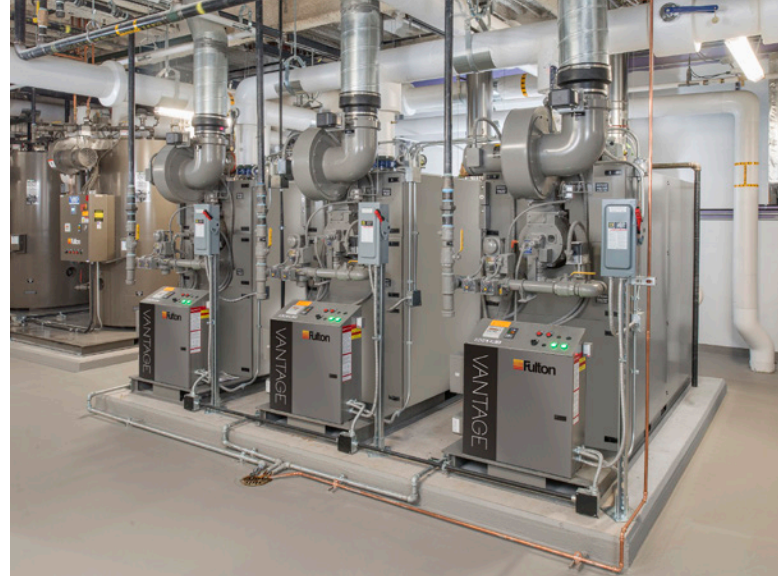
▲ A healthcare facility in Wisconsin utilizes three Vantage 3.0 MM BTU/hr boilers for multiple heating applications
